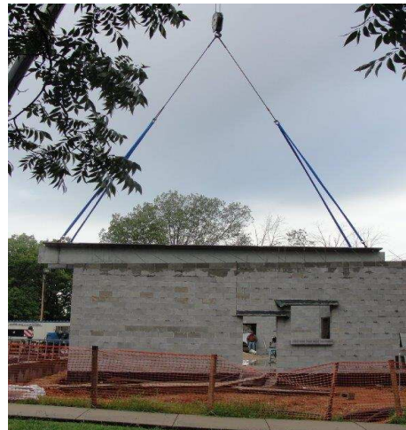
(Right) Construction of Community Safe Room.
